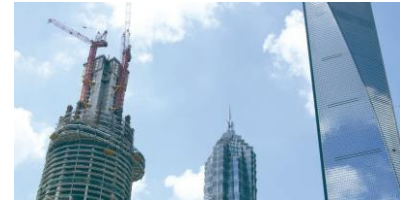
Upon its completion, the Shanghai Tower (left) will be the tallest building
