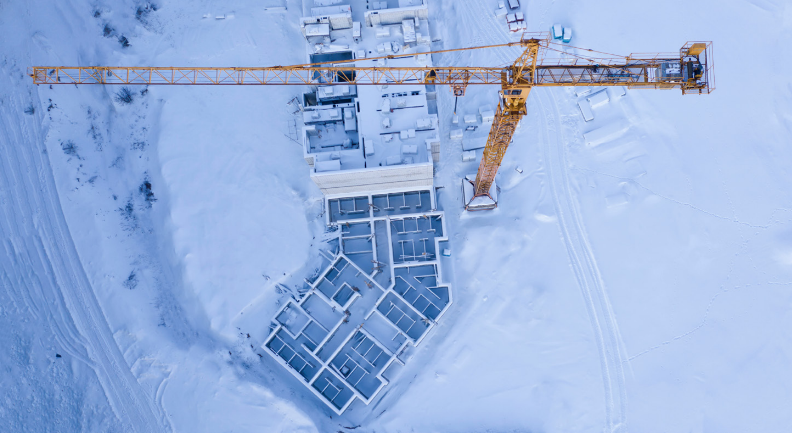
Snowy, abandoned, empty construction site. Credit: maykal/Adobe Stock
