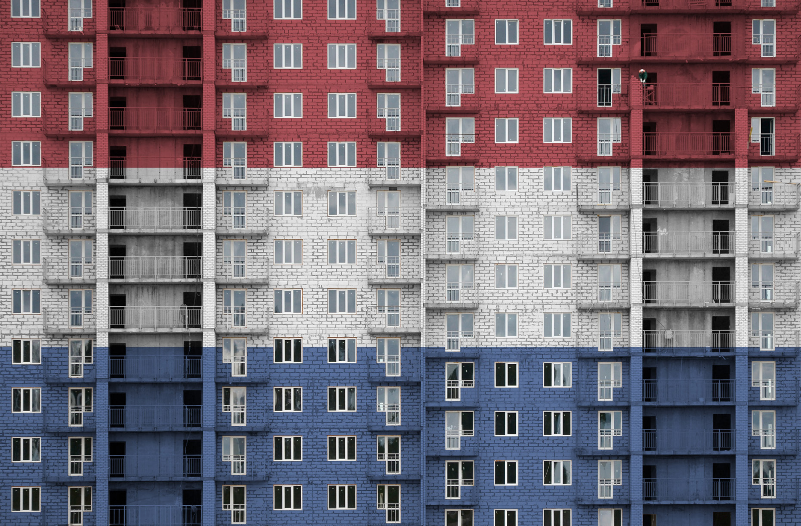
Netherlands flag depicted in paint colours on a multi-storey residential building under construction. Credit: mehaniq41/Adobe Stock
