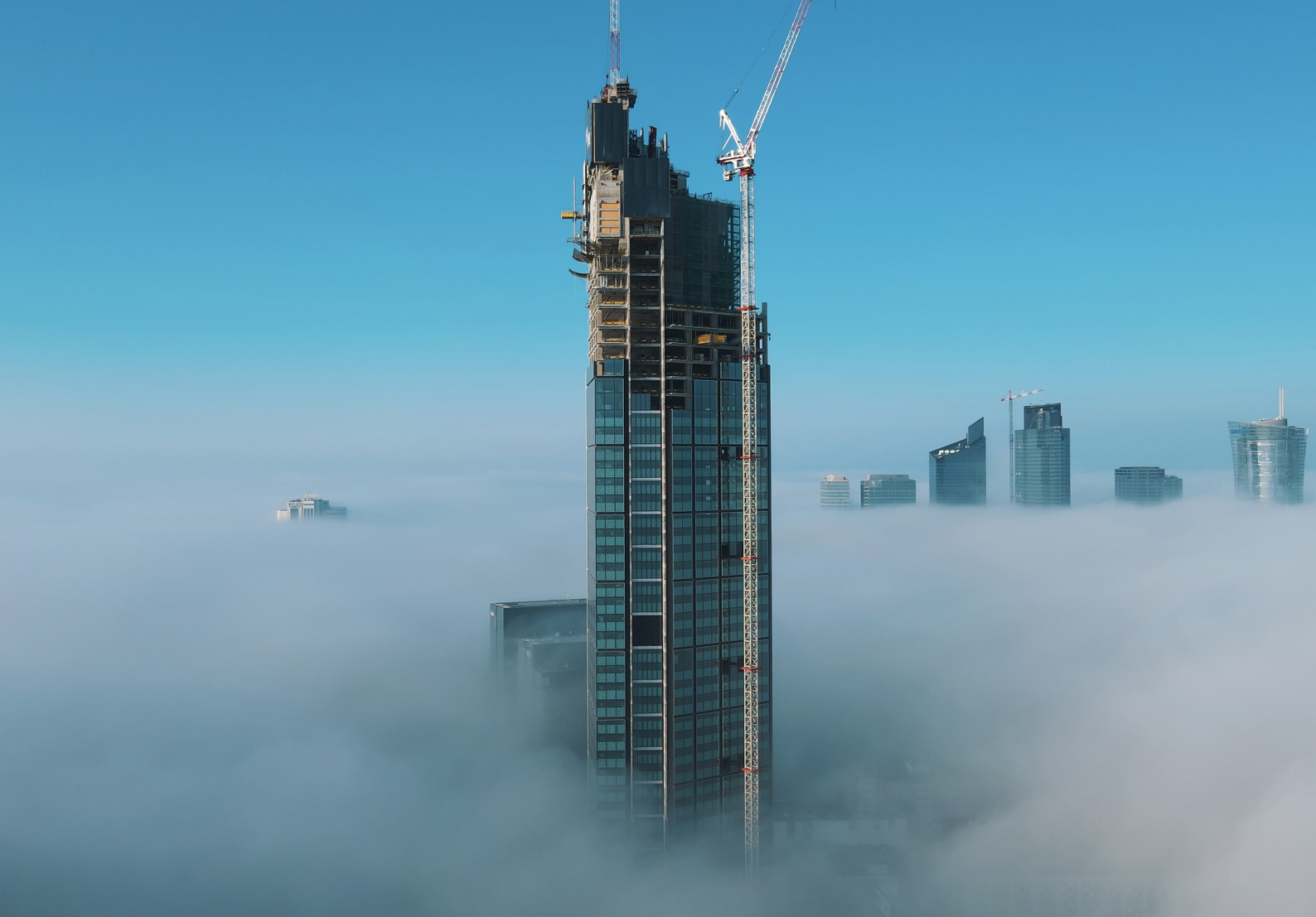
Varso Tower under construction rising above clouds, Warsaw, Poland. Credit: CameraCraft/Adobe Stock
