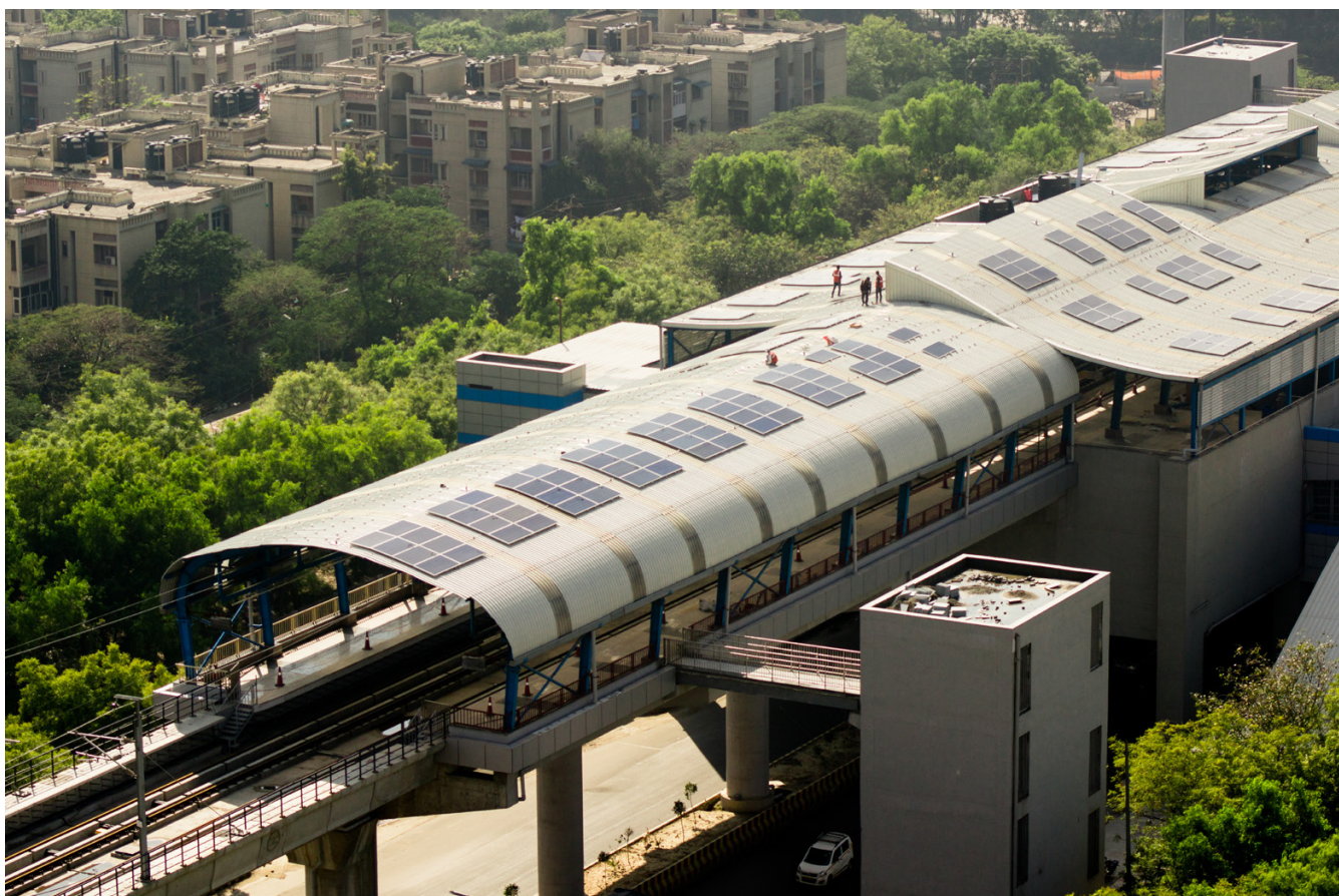
Aerial shot of Delhi metro station with solar panels being installed. Credit: Memories Over Mocha/Adobe Stock
