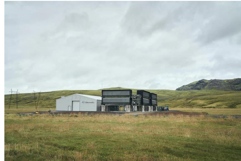
First commercial Direct Air Capture Plant (DAC) in Iceland
