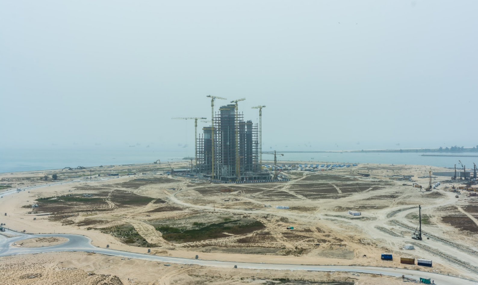
Eko Atlantic City under construction in Lagos, Nigeria. Credit: MOdAMO/Shutterstock
