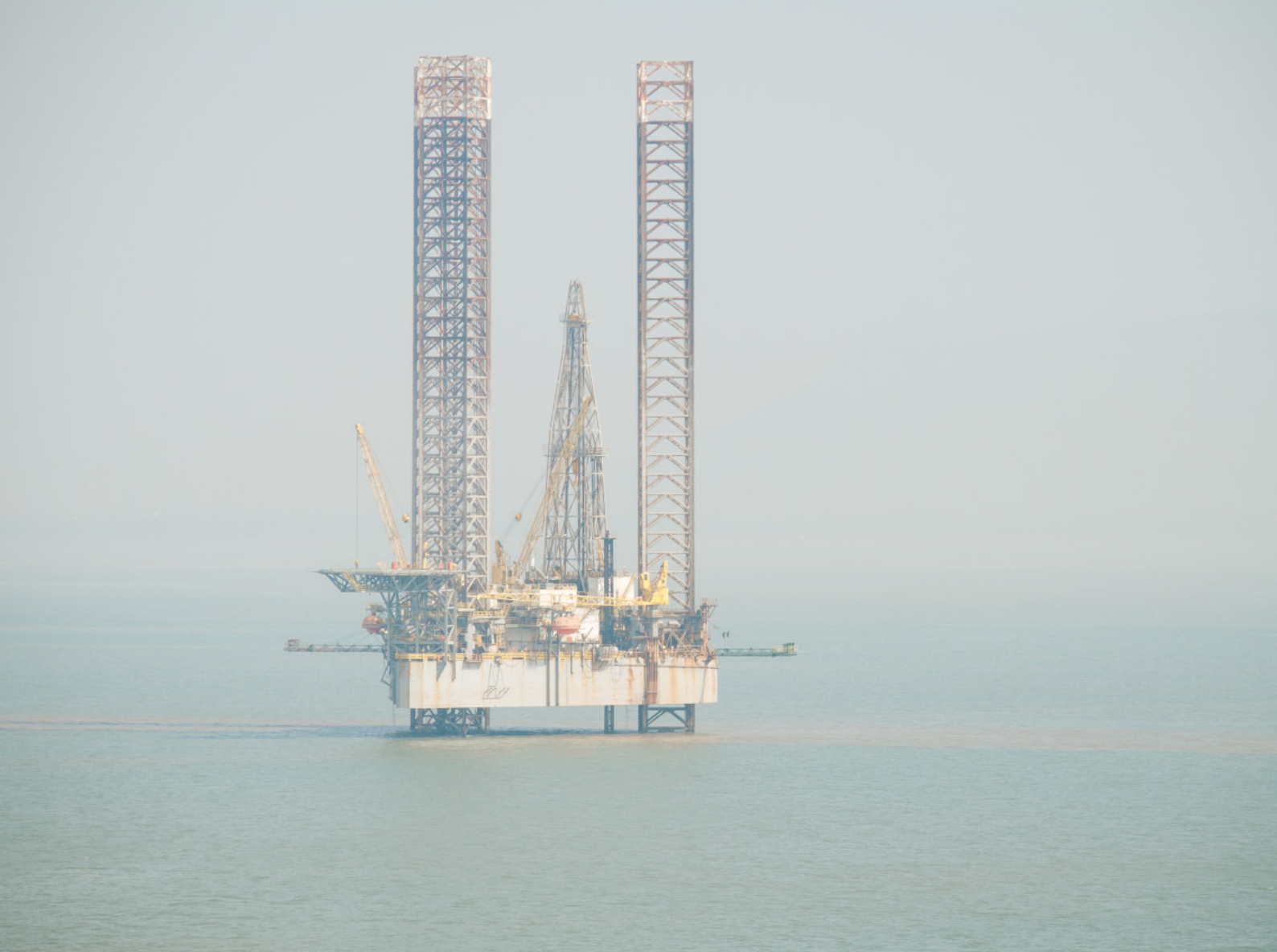
Offshore jack-up drilling rig and gas production platform in Indian waters. Credit: Jevgenijs/Adobe Stock
